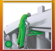
Correct – use of a stand-off device to ensure a strong resting point. Do not rest a ladder against weak upper surfaces
