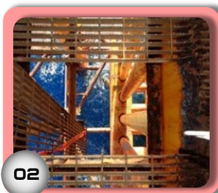
Post-Incident photograph of hazardous grating section suspended in open hole
