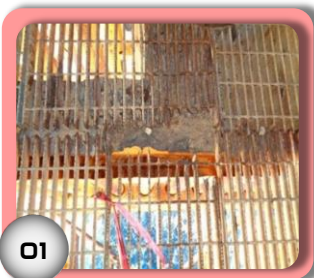
Pre-Incident photograph of hazardous grating section
