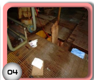
Post-Incident Photograph of hazardous grating section
