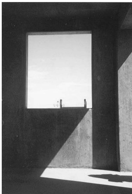
FIGURE 25.3 Forty-two inch window sill and ladder tip. (Photo from NIOSH.)
