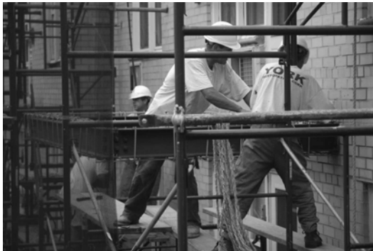
FIGURE 27.2 Construction workers using scaffolding on the side of a building.
