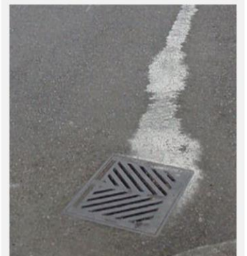
Storm Drains- Frequently check hydraulic lines for trash compacters that are
