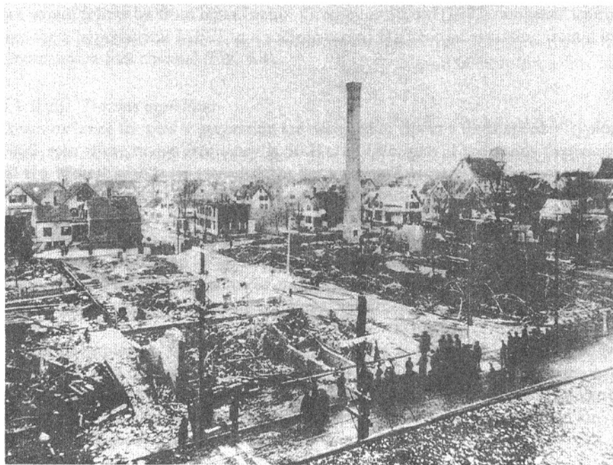
Fig. 5.2 A boiler pressure vessel exploded in a factory in Massachusetts in 1905. There were 58 fatalities (photos courtesy Hartford Steam Boiler Inspection & Insurance Company)
