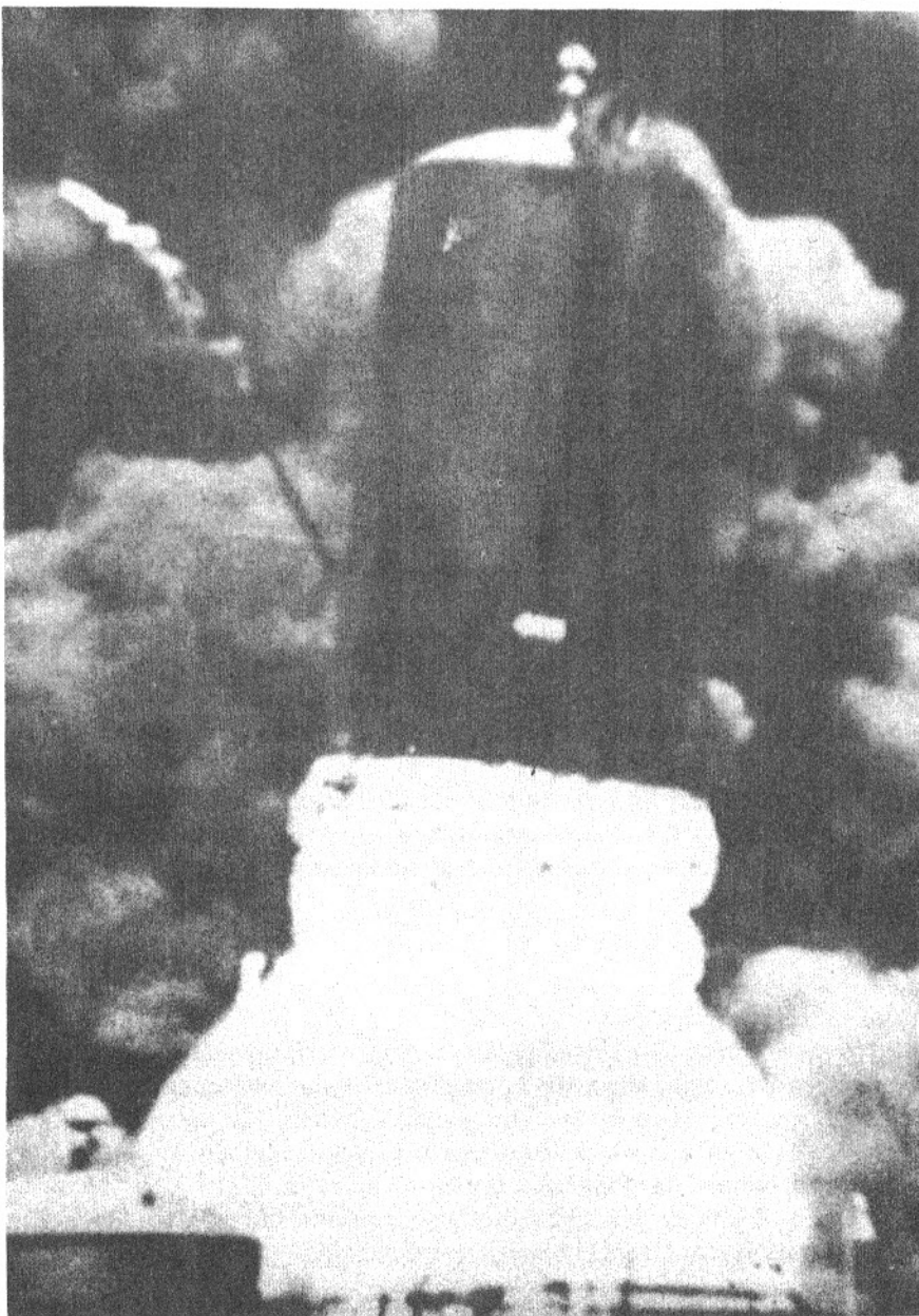
Fig. 5.1 In Boiling Liquid Expanding Vapour Explosions (BLEVEs), the storage tank normally ruptures and a 'fireball' explosion ensues. In this case in New Jersey in 1949, however, the tank, containing 106 T of hydrocarbon, rocketed a distance of several hundred metres. There were four fatalities (photo courtesy NFPA)
